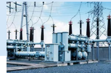
发电站 POWER PLANT
